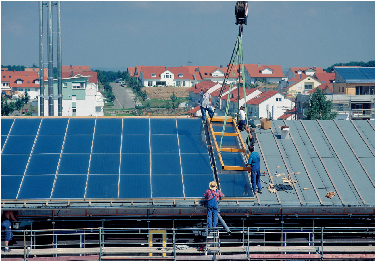
Figure 2: Construction workers installing PV systems (Source: MEV Verlag GmbH)
