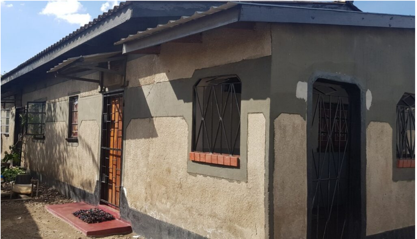
Figure 1: A house built with concrete blocks with cement/mud plaster.
