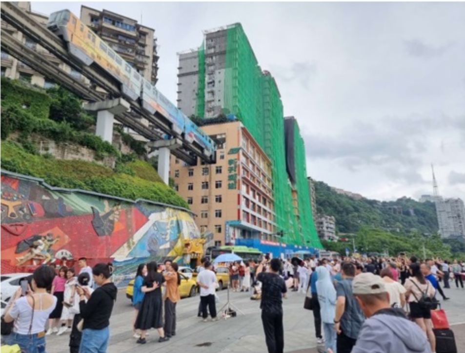
Figure 3 Liziba (李子坝) Metro Station
