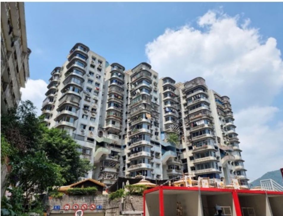
Figure 1 Baixiangju (白象居) Residential Building
